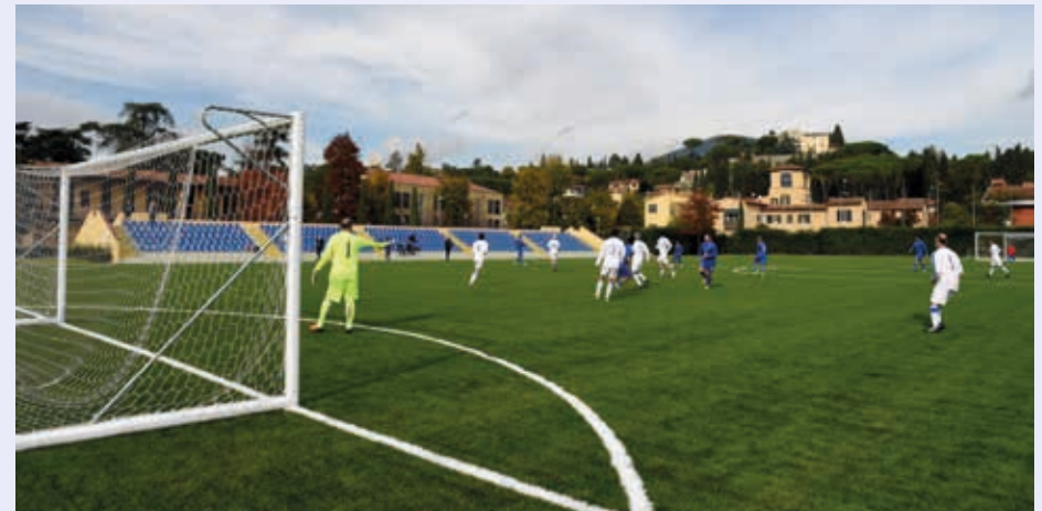
The new pitch 1, made with the latest generation artificial turf. The uncovered stand was also rebuilt and now has 350 seats.
