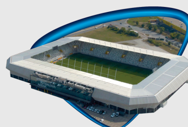
KOSICE FOOTBALL STADIUM
